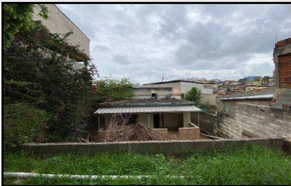
CASA PRINCIPAL - TERRENO DECLIVE
